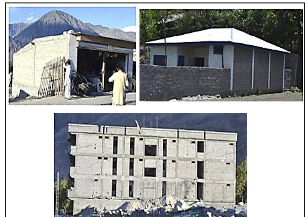
Figure VIII: Concrete Masonry (CM) Building with Flat Corrugated Roof; Concrete Masonry (CM) Building with Corrugated Pitched Roof; Reinforced Cement Concrete Building [11]
